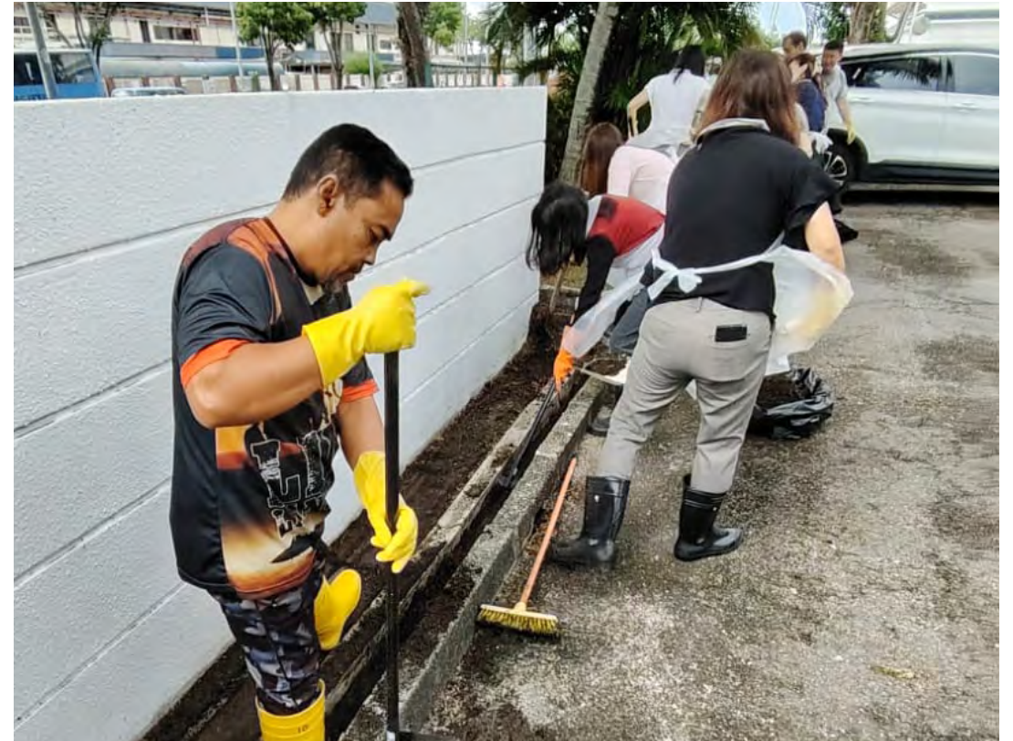
Drainage cleaning near the plant by employees (Penang FIZ3 Site)
