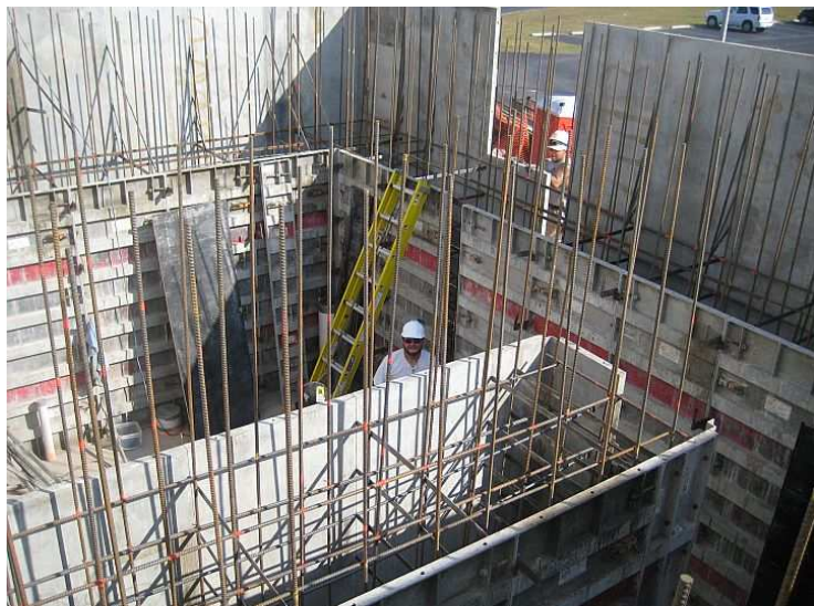
Fig. 5: View of wall forms before the second (wall) concrete pour. The labyrinth vault access architecture can be clearly seen.
