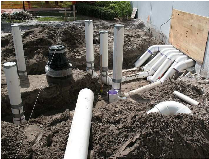
Fig. 4: Site excavation before pouring the vault foundation. The top of the source well is clearly visible to the left of image center. The PVC piping provides cable raceways between the vault and the Intersil Palm Bay building 58 control room (right).
